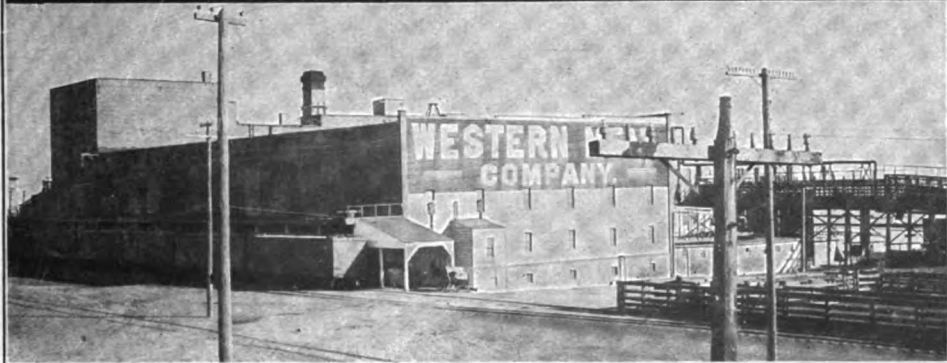
1—Plant of the American Jupiter Steel Company. 2—Gas Tanks of Electric Power Plant. 3—Powerhouse San Francisco Gas and Electric Company. 4—Plant of The Western Meat Company
